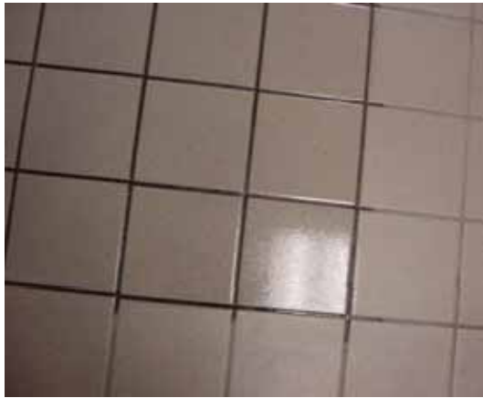
Glazed Tile Bathroom Winn Dixie Distribution Center
