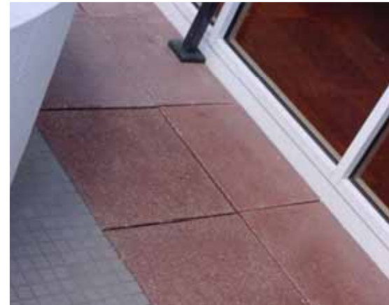
Tinted Concrete Grand Hotel – Pool Deck
