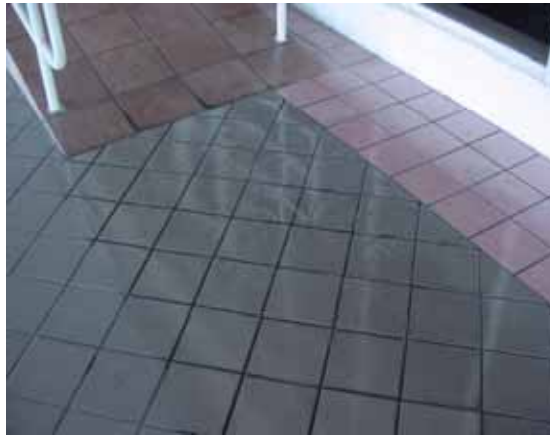
Polished & Quarry Tile Walkway Grand Hotel & Condo-Miami
