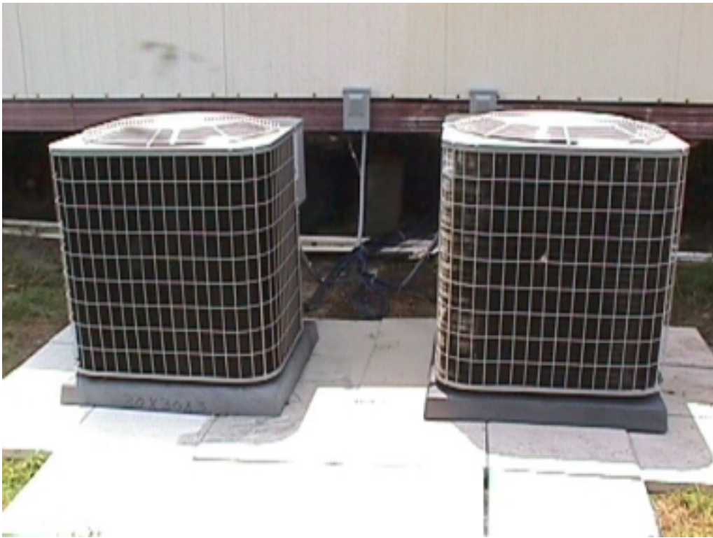
Figure 1. Installation of Two Carrier Condensers Side by Side for Test. Unit B1, the Adsil Unit Has Been Cleaned and Some of the Black Factory Coating Removed.
