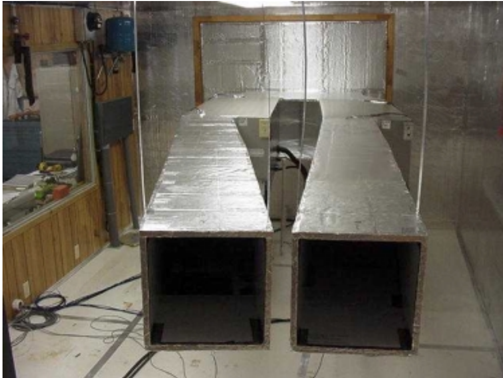
Figure 5. Side by Side Installation of Air Handlers within Appliance Laboratory.
