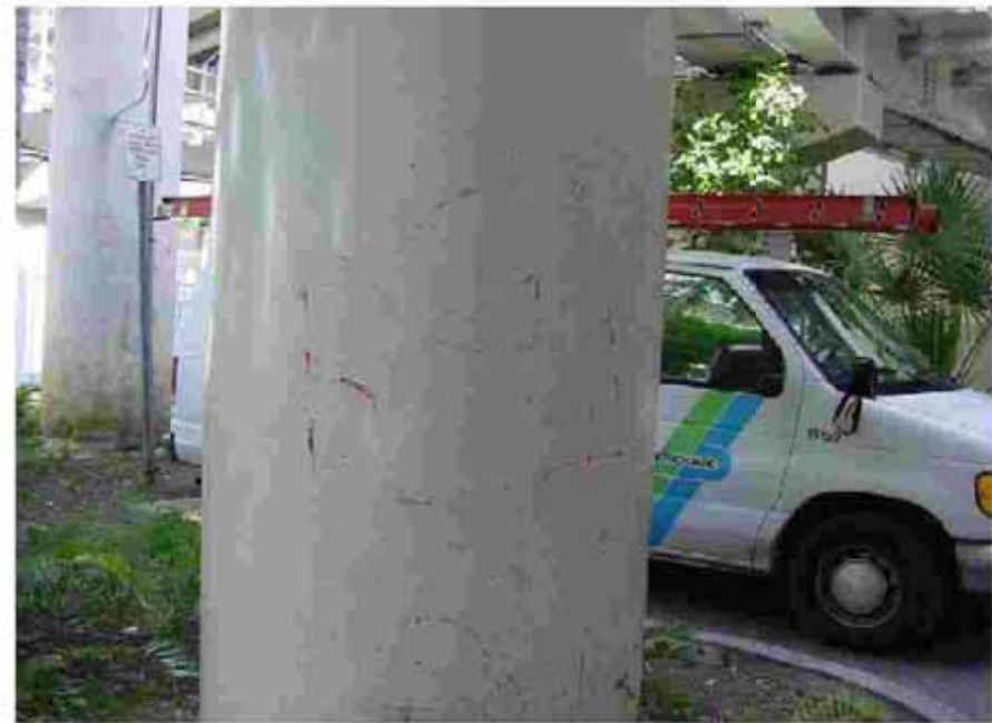
Complete Graffiti Cleaning with AD1-919... ( Scrub brush needed for cracks in cement )
