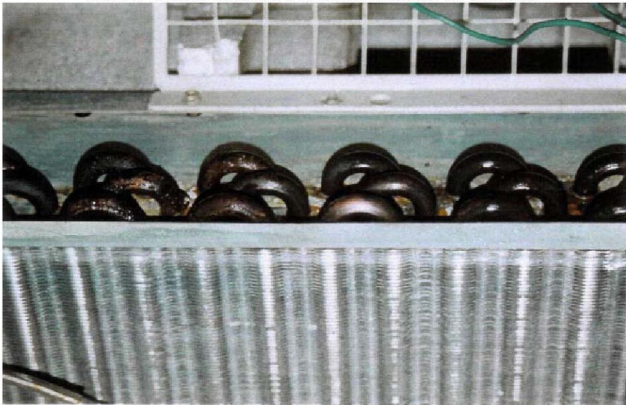
Below Photo: Coated with ADSIL after 24 months
