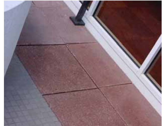
Tinted Concrete Grand Hotel – Pool Deck
