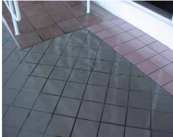
Polished & Quarry Tile Walkway Grand Hotel & Condo-Miami
